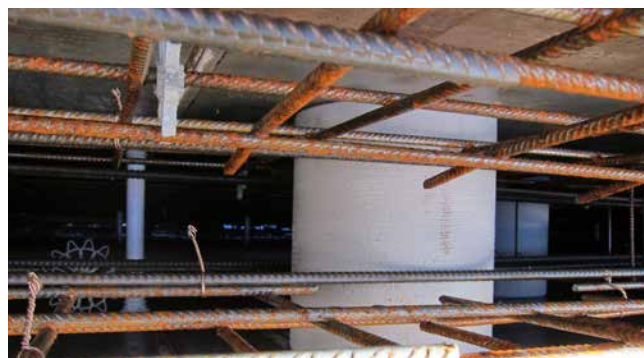
ZVR200/300 in de bekisting vastgezet
